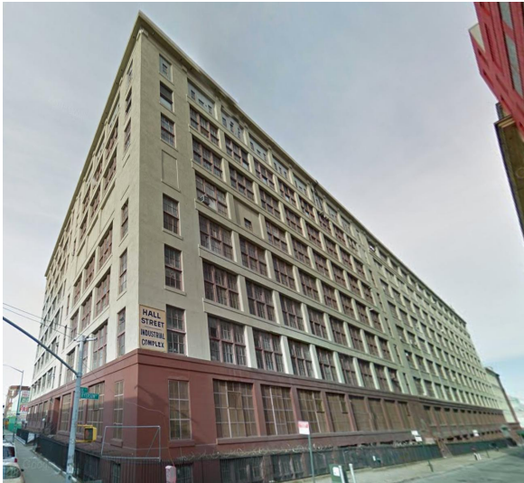
The highest priced industrial/office sale was 39-43 Hall Street in Clinton Hill, which sold for approximately $161M in March. The property contains approximately 547K SF.
